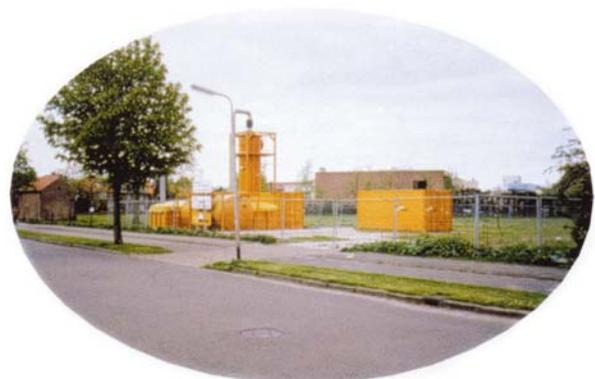
***On-site treatment of groundwater pumped from an aquifer contaminated by chlorinated hydrocarbons.***
